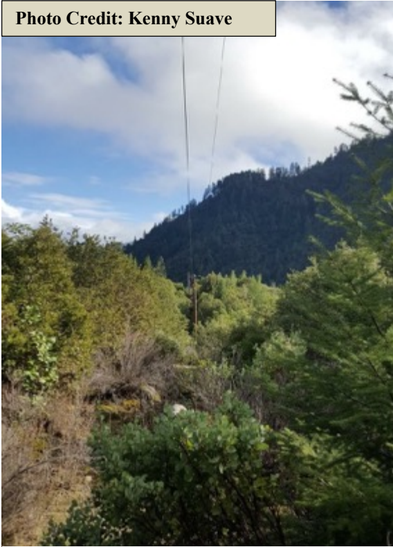
Figure 5.3 Even Maintained Corridors Have Unsafe Levels of Fuels Near Lines
